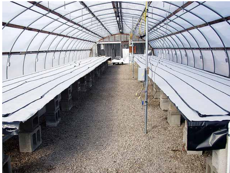
Figure 7. Setup of the CapMat II fertigation system. The black emitter strips are shown. The reflective mulch was placed over the CapMat fabric.
