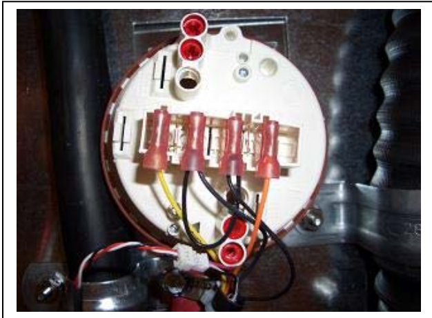
Figure 11 Above: Fill Trap Switch. Fill Switch has replaced traditional Float Switch in the new style Steam & Flask Scrubber Glassware Washers. Fill Switch may be referred to as the “pressure switch”.
