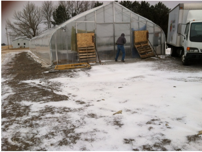
Figure 2. One problem with high tunnels versus greenhouses is the lack of insulation. Here Ryan used pieces of plywood to temporarily seal off the vents on the outside and old comforters on the inside.
